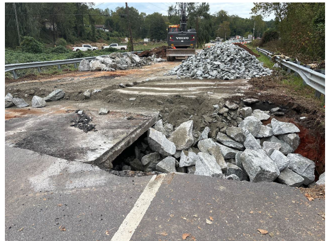
Flood waters induced by Helene's rainfall washed out this section of U. S. Highway 276 (Geer Highway) just west of Cleveland.
